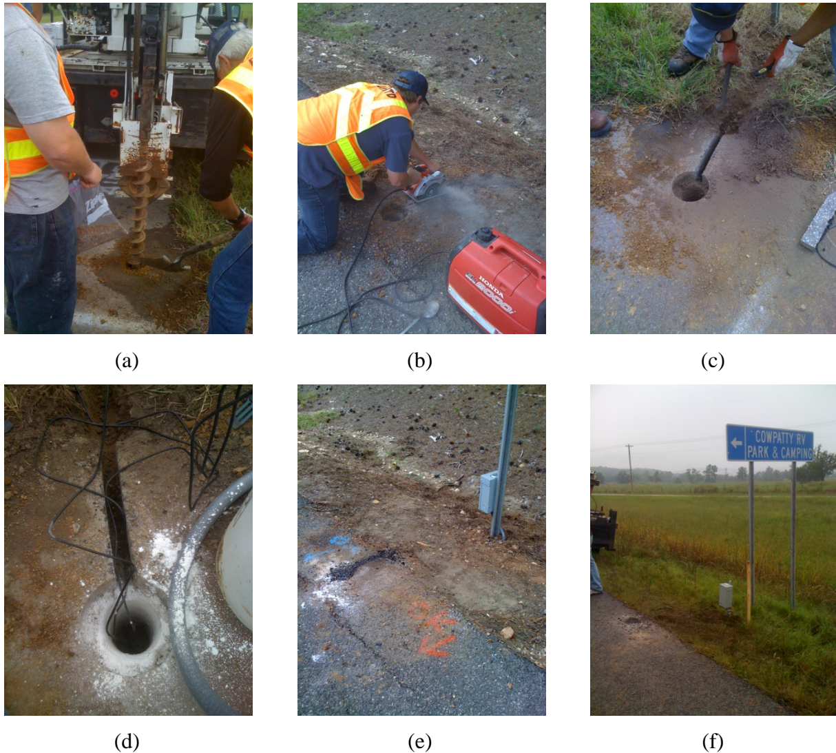
Figure 4.5: Field monitoring system installation pictures: (a) Auguring through base course; (b) Creating channel through asphalt; (c) Final channel in asphalt running to the edge of the shoulder; (d) installation of sensors and backfilling with silica flour; (e) Cold-mix patch on surface; (f) Datalogger box in shoulder attached to metal post
